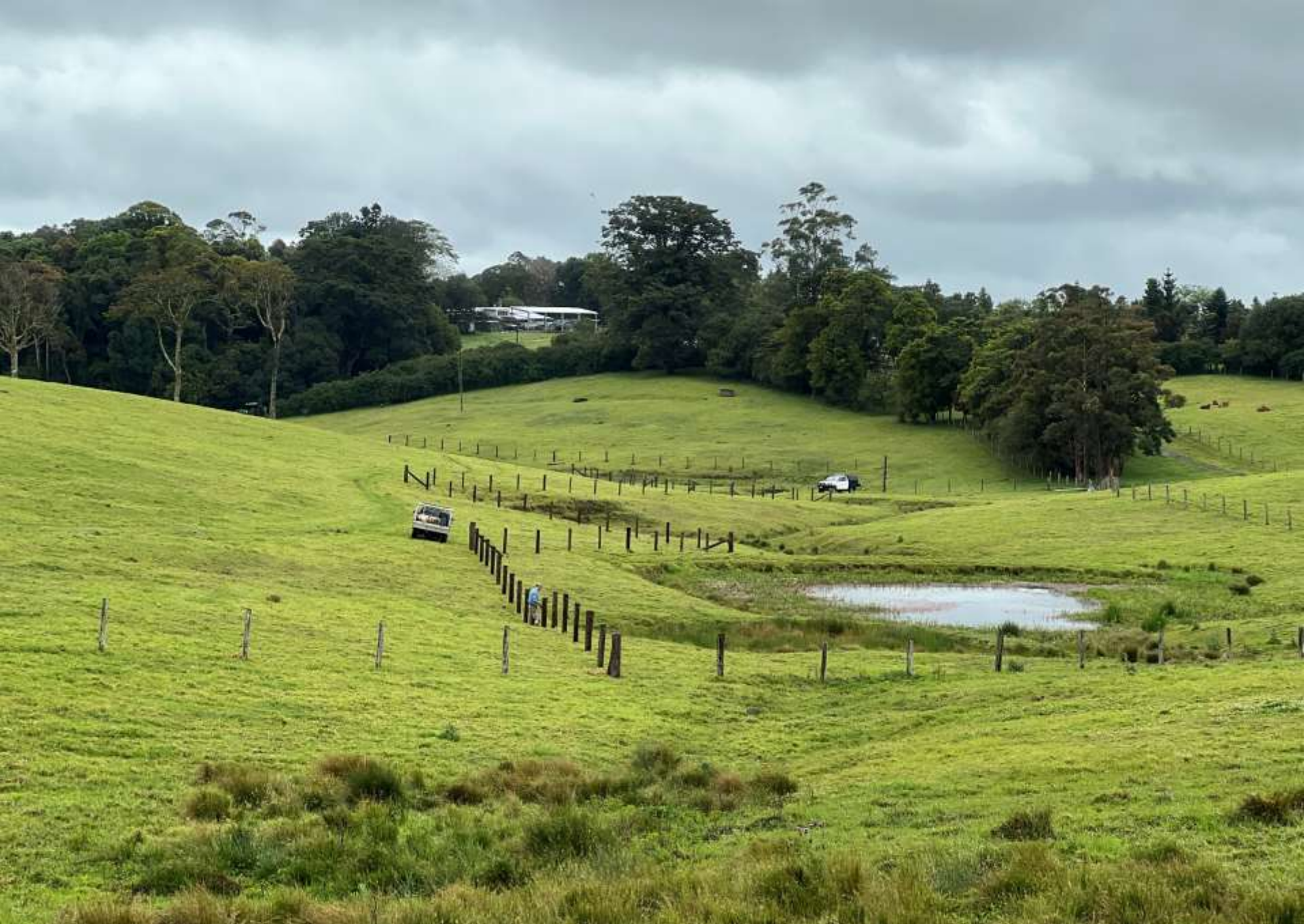
Fencing has begun on the Daley Farm with Tag Rural Fencing
