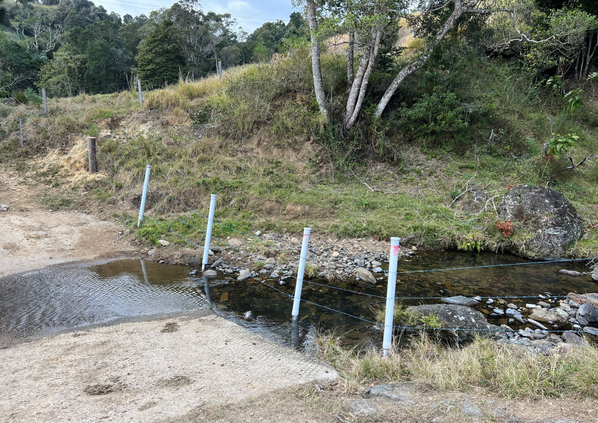
Currently trialling a new flood fence design on Alcorn Creek
