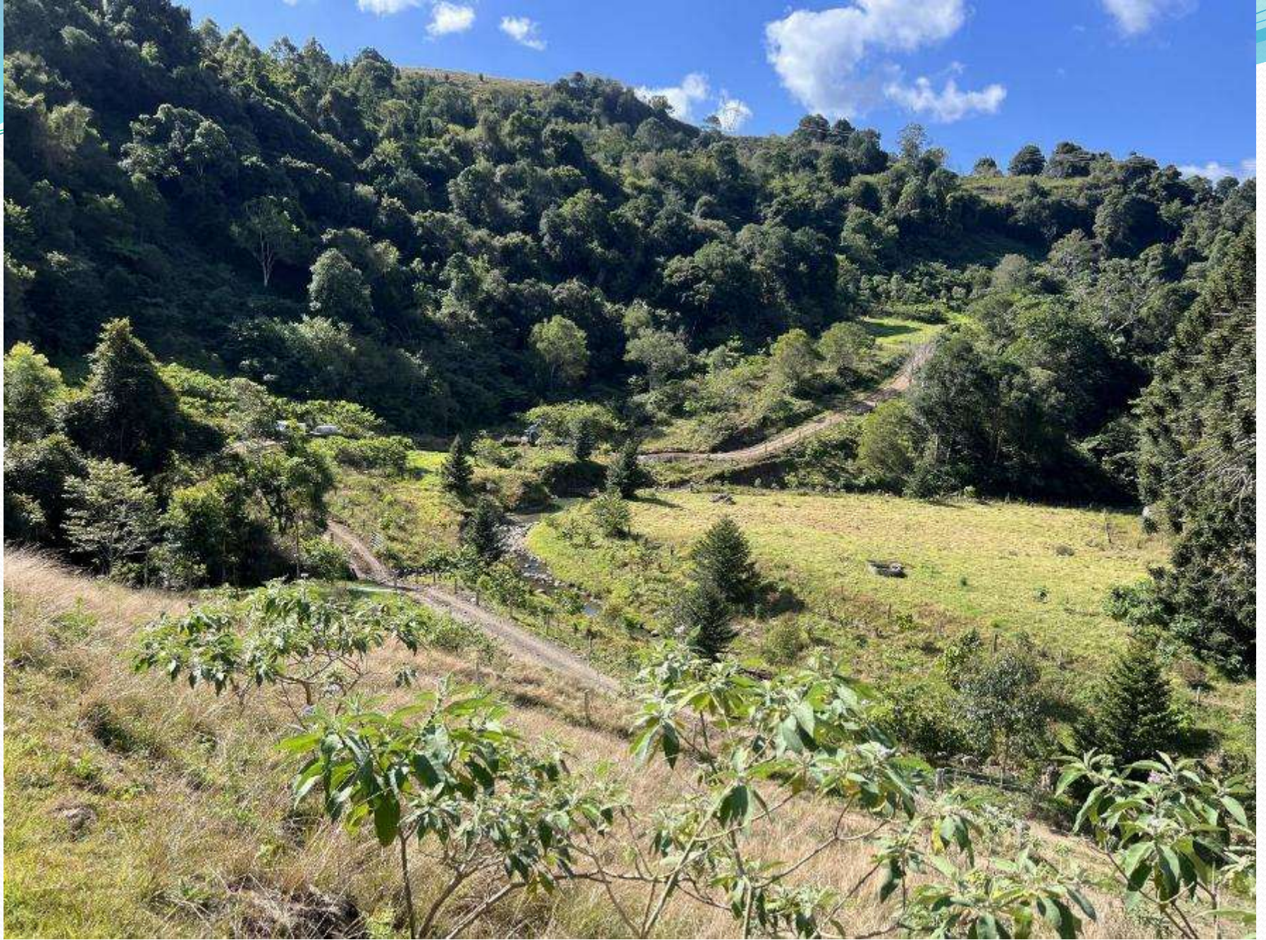
250 m of new access track has been installed
