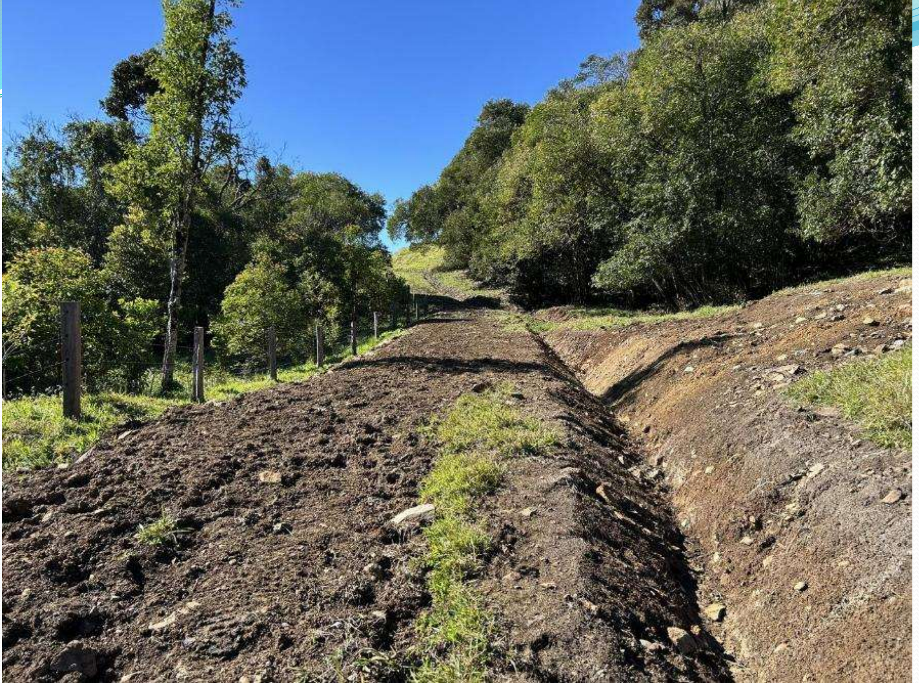
Redirecting overland flow of water, preventing it from further destabilising the site
