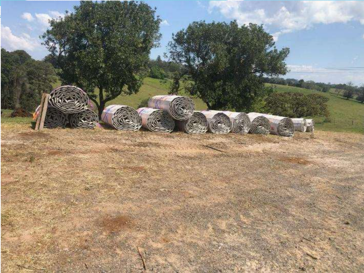
Manager assisting with short term storage of concrete mats
