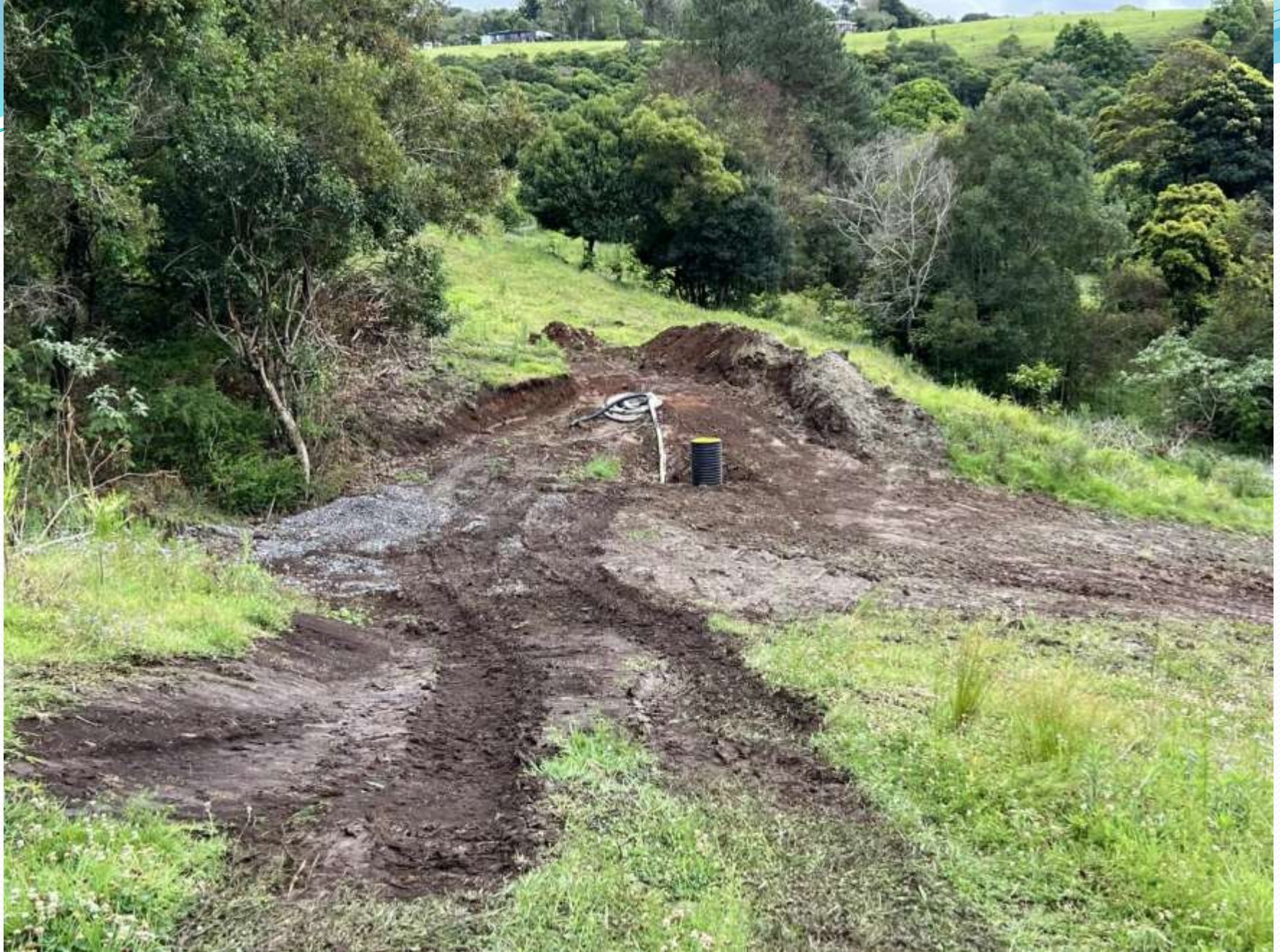
3 Wells to be installed, one completed
