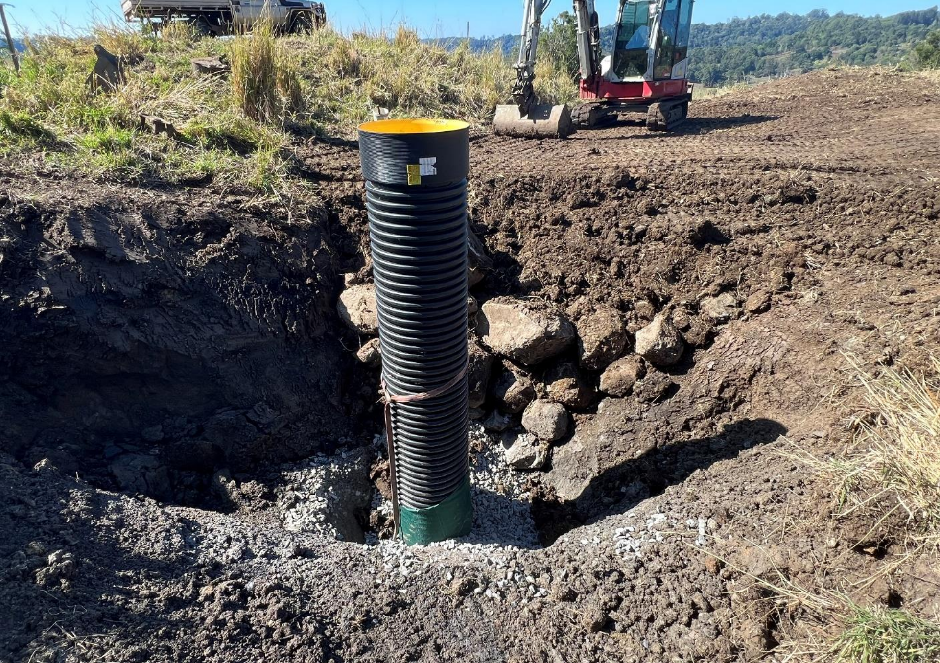
Final well insulation on the Crick Well Project
