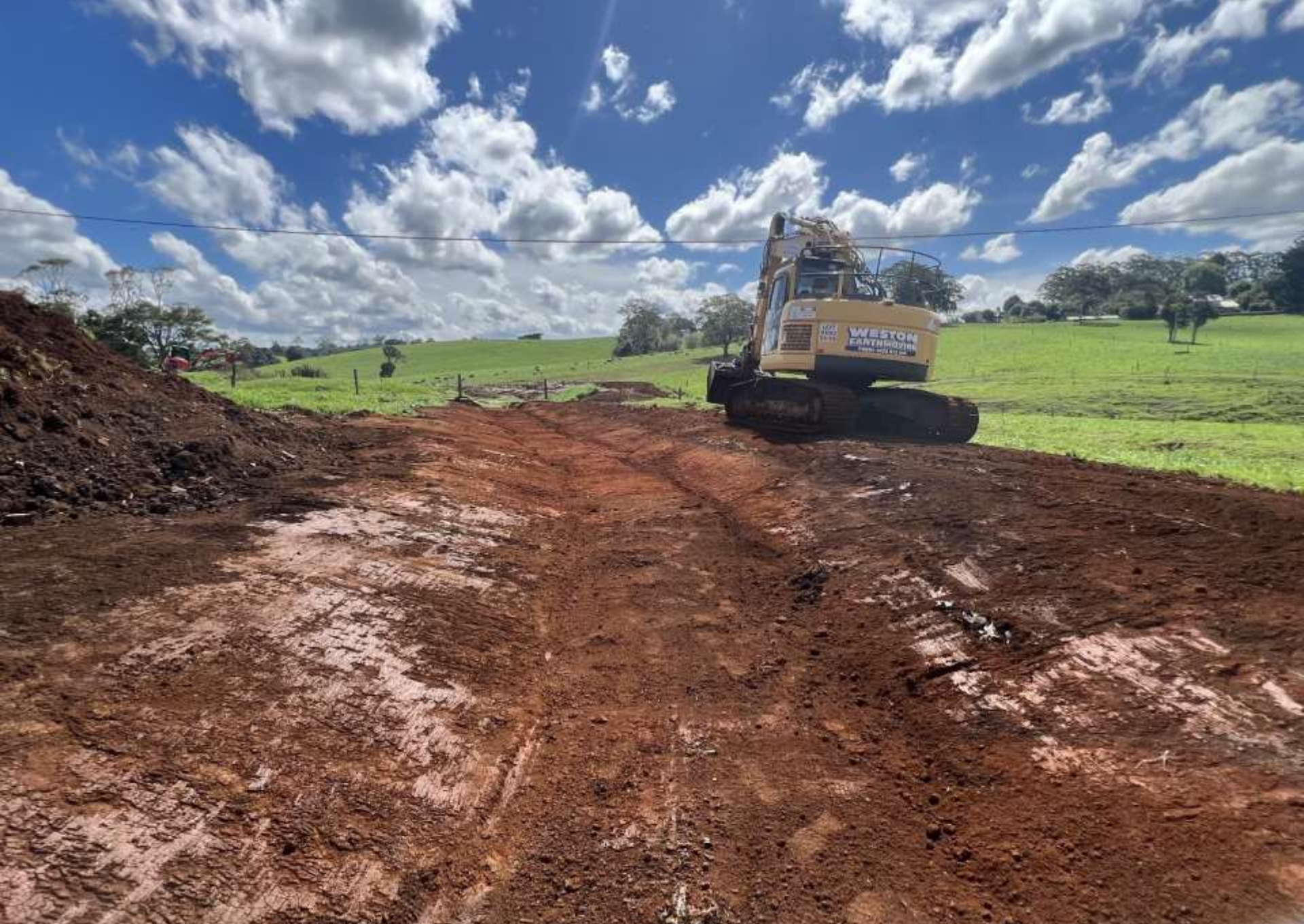
• 50 meter contour drain connecting feed pad to the effluent pond
