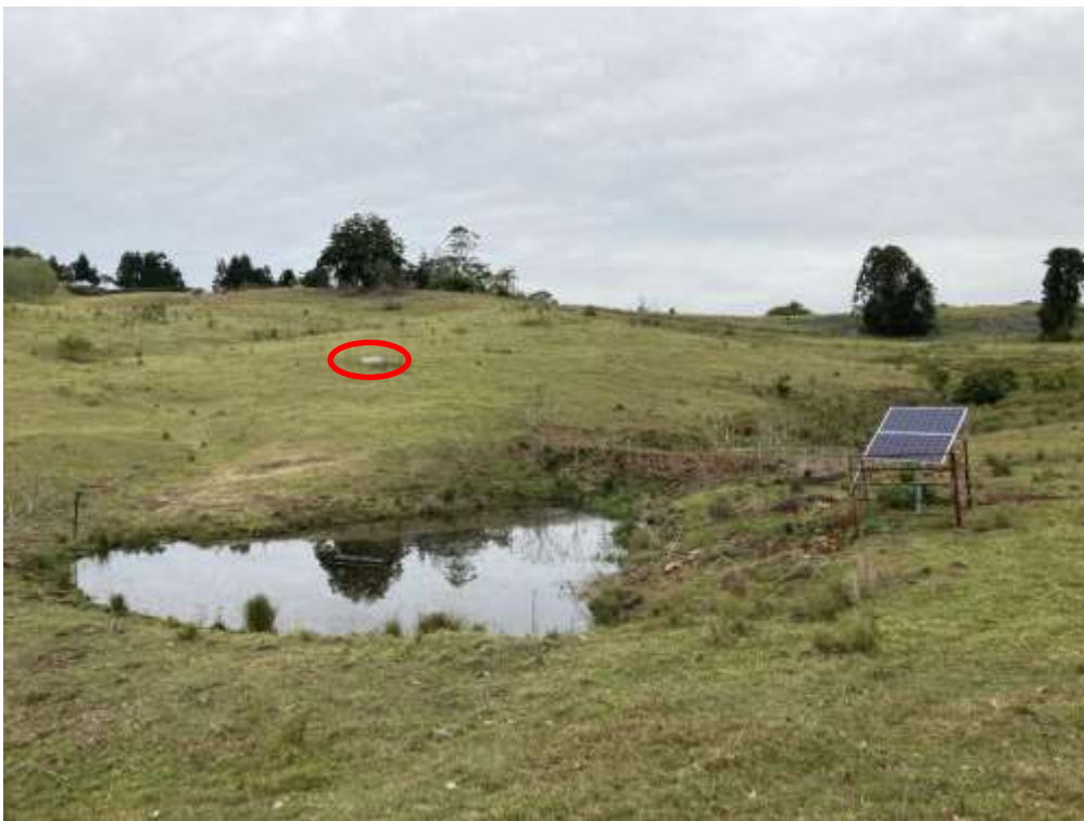
Above: The solar pump installed, which lifts water to a header tank. The water is then gravity fed to four water troughs. A trough is highlighted that will provide water for livestock, following the fencing of the riparian zone.
