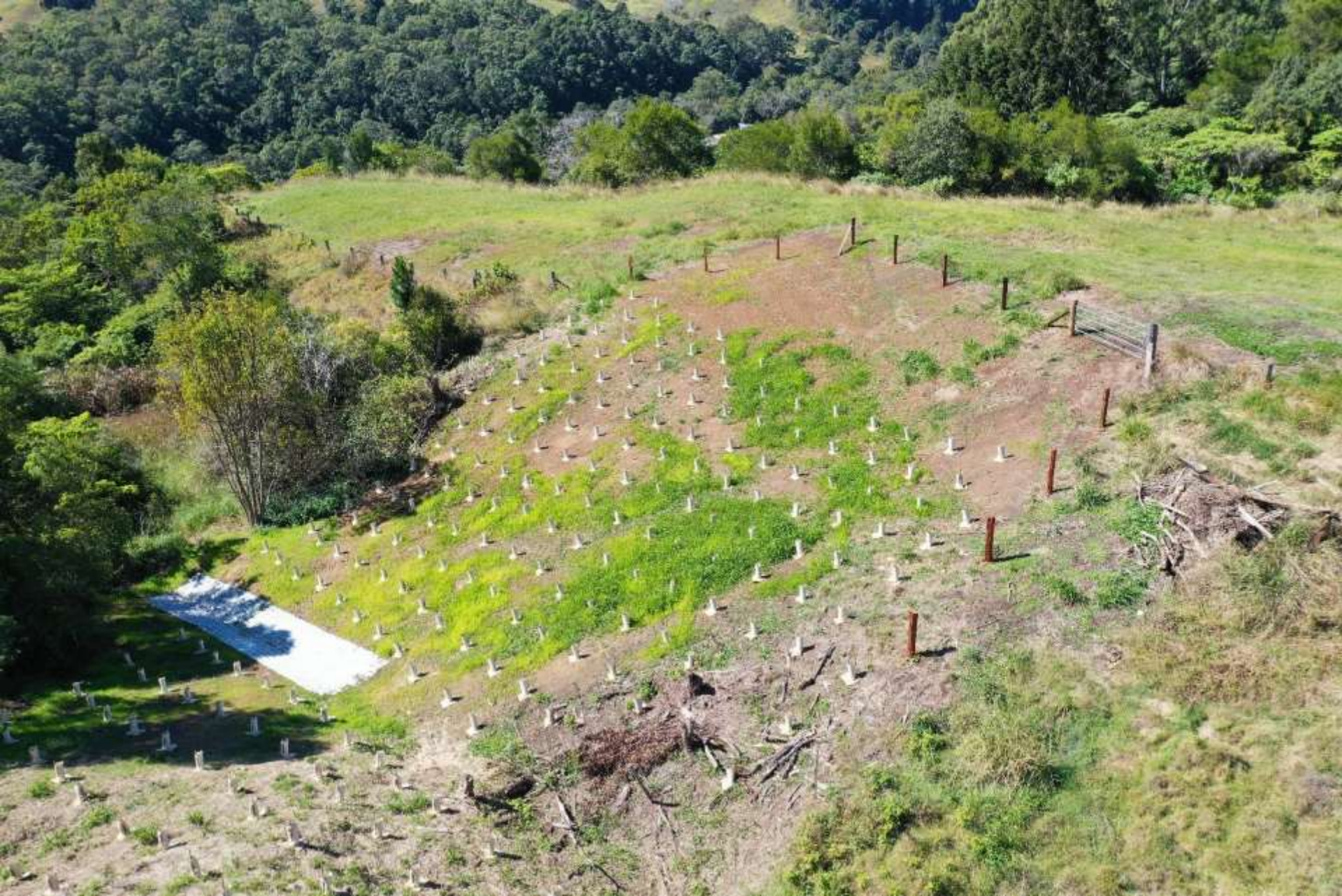
Landslip Site – Fenced, subsurface drainage, concrete matting and revegetation (350 stems)
