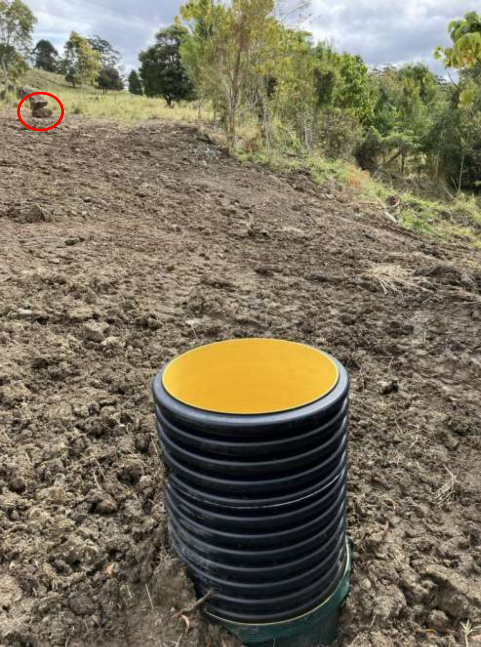
Well 2 - Completed with subsurface drainage running to the two rocks
