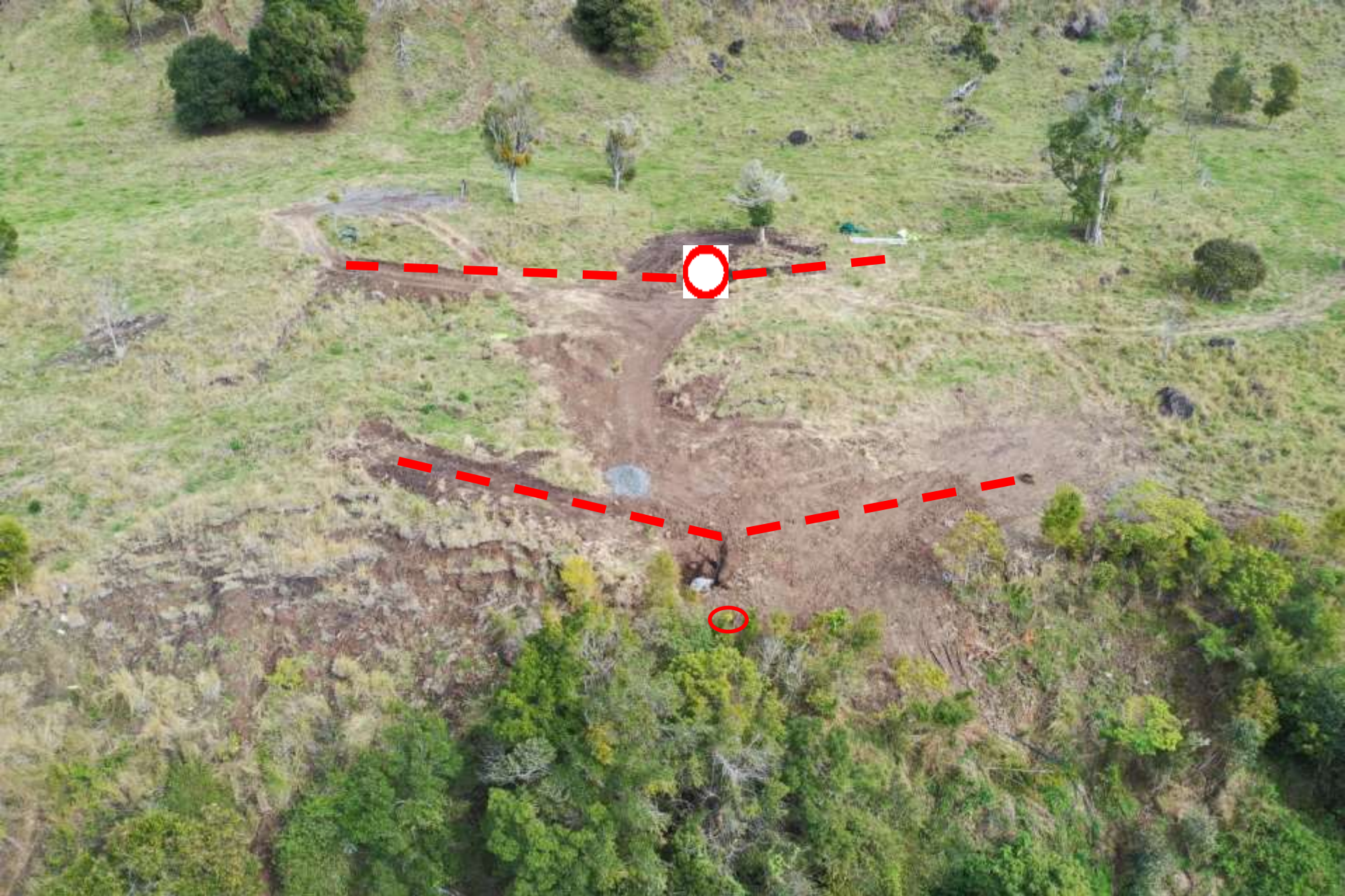
Site 2 – Wells installed, further subsurface drainage to be completed.
