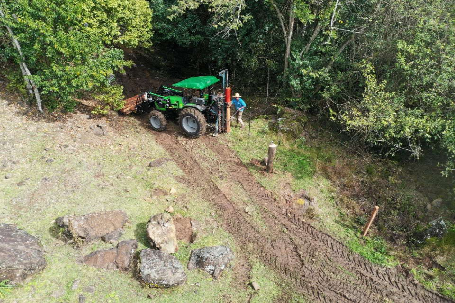
Creek fencing – 900 m
