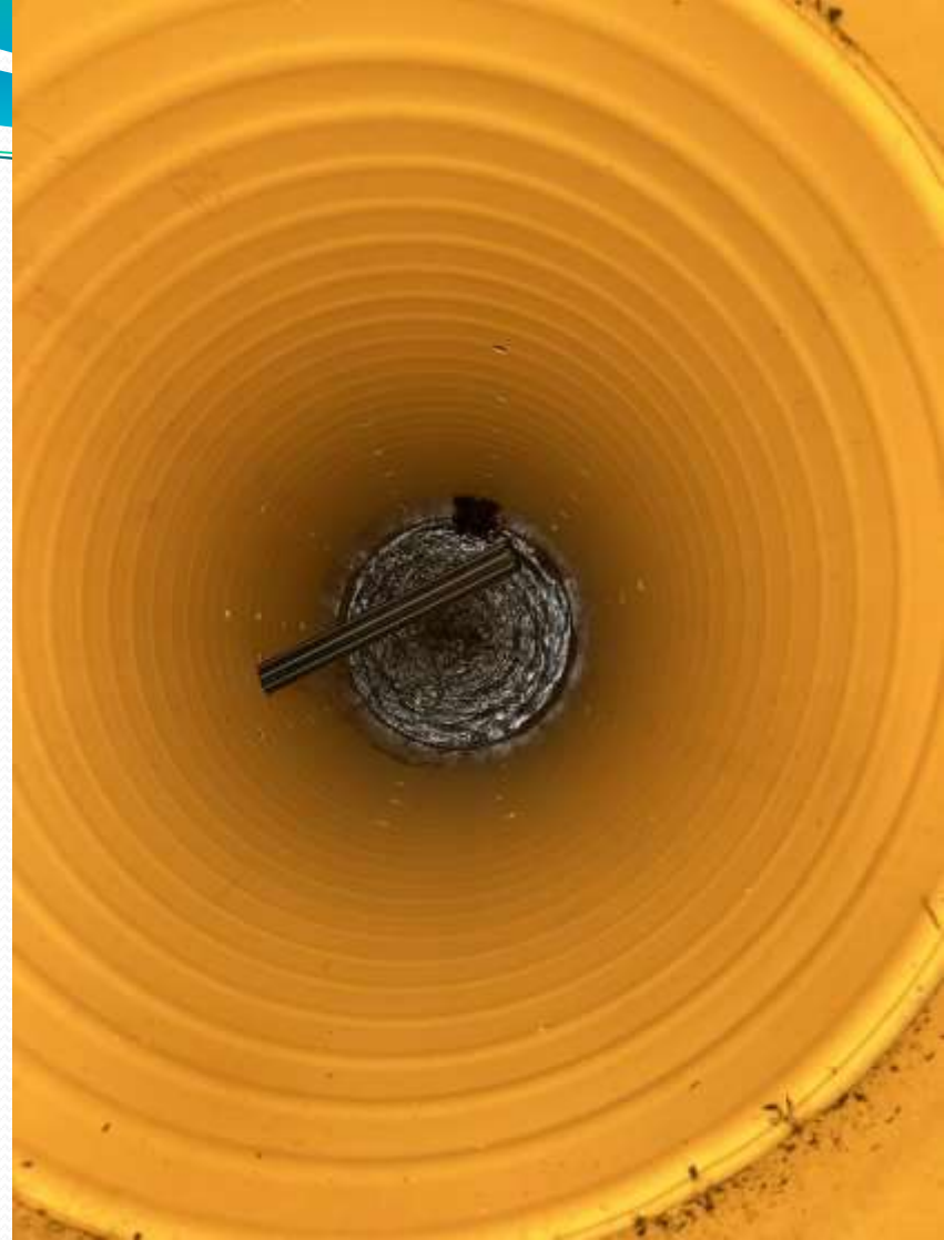
Water running in from the top well Site 1: 3,927 L/Day Site 2: 1,353 L/Day
