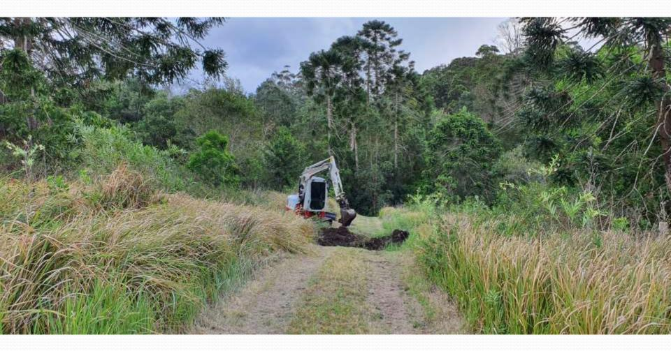
Nash Excavations placing drainage pipes in access tracks
