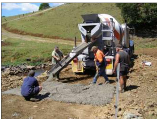
Low level concrete crossing construction
