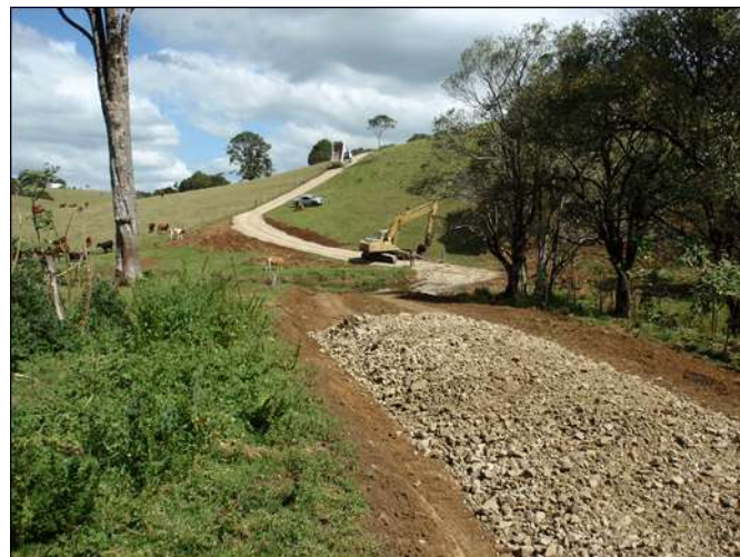
Laneway construction utilising locally sourced road base
