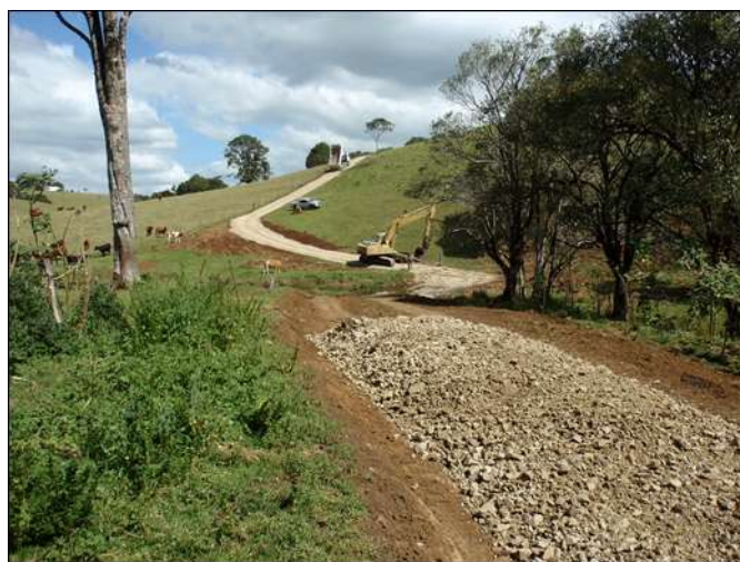
Laneway construction utilising locally sourced road base
