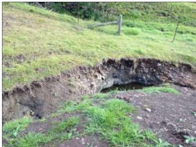
Head-ward erosion threatens the dam wall. The dam is critical for the off stream watering infrastructure. Dam wall failure can result in a significant delivery of sediment to catchment waterways
