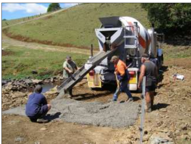
Low level concrete crossing construction
