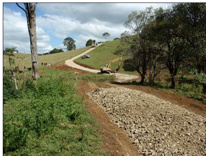
Laneway construction utilising locally sourced road base
