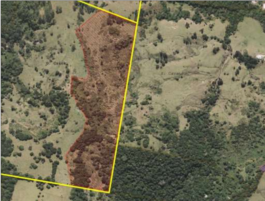
Figure 1: The Crick property on the left with the very unstable Cavanagh property on the right. The shaded area is the focus of this project – weed management, improved livestock management and preparation for the 2015-16 Seqwater Landslide Remediation program.
