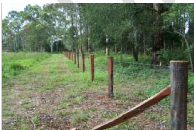
Above: Standard cattle fencing will be installed. A top plain wire will be installed (if possible) to minimise interference with wildlife.
