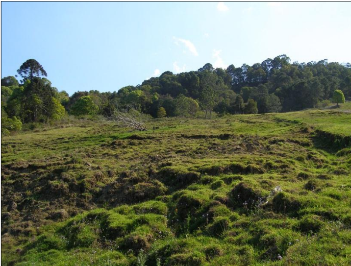
Above: Landslips are difficult to revegetate, however the area to the right of the figure is stable and can be reliably planted to commence stabilisation.
