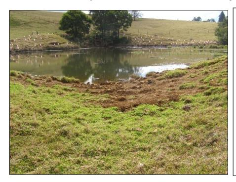
Left: The overflow of the main dam. This area is main waterway the crossing to the south western paddocks of the property. In wet periods this crossing is damaged stock with the resultant sediment and nutrients travelling a short distance to the Obi Obi Creek.
