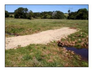
Left: The waterway crossings constructed in previous projects have been effective, however road base material is required to extend the hardened surface to reduce the amount of 'pugging' leading up to the crossing.
